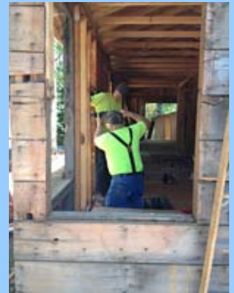
Walt, Connor & guys got the framing done!
